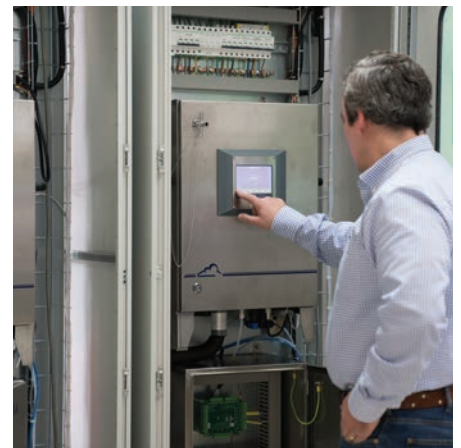
GAS ABATEMENT MONITORING OF MULTIPLE GASES
