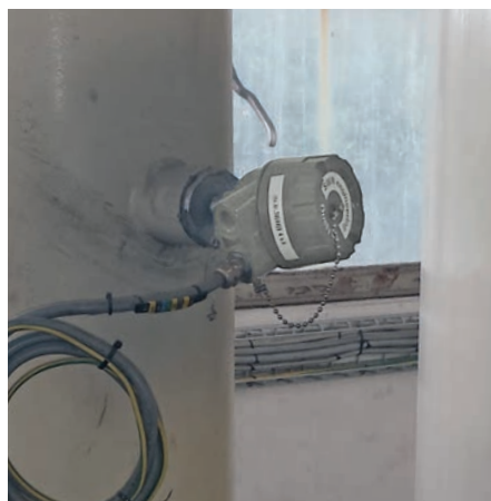
COMPACT SENSOR FOR BROKEN BAG DETECTION
