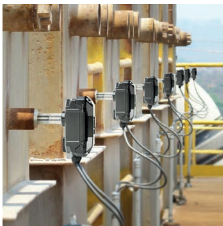
BROKEN BAG DETECTION WITH EXTERNAL DISPLAY
