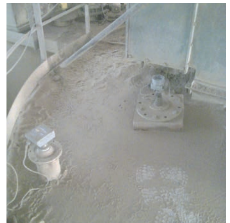
INSTALLATION FOR LEVEL MEASUREMENT IN SILOS
